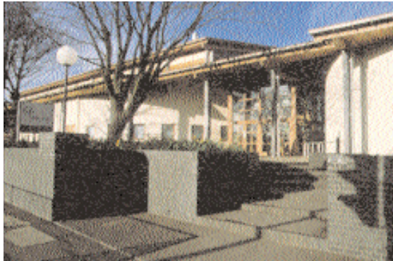
An inviting, recessed entrance provides a welcoming introduction to a sports centre.
